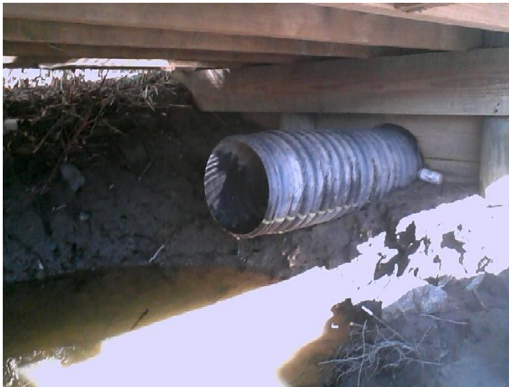
SLHDPE (Smooth-Lined High-Density Polyethylene):
